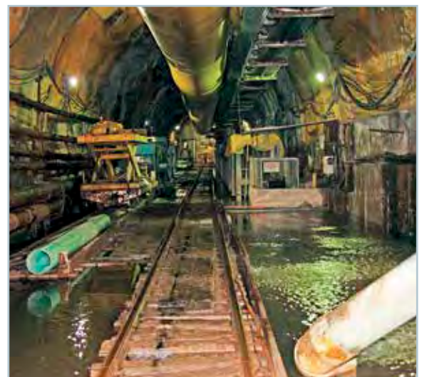
Intake No. 3 Construction
